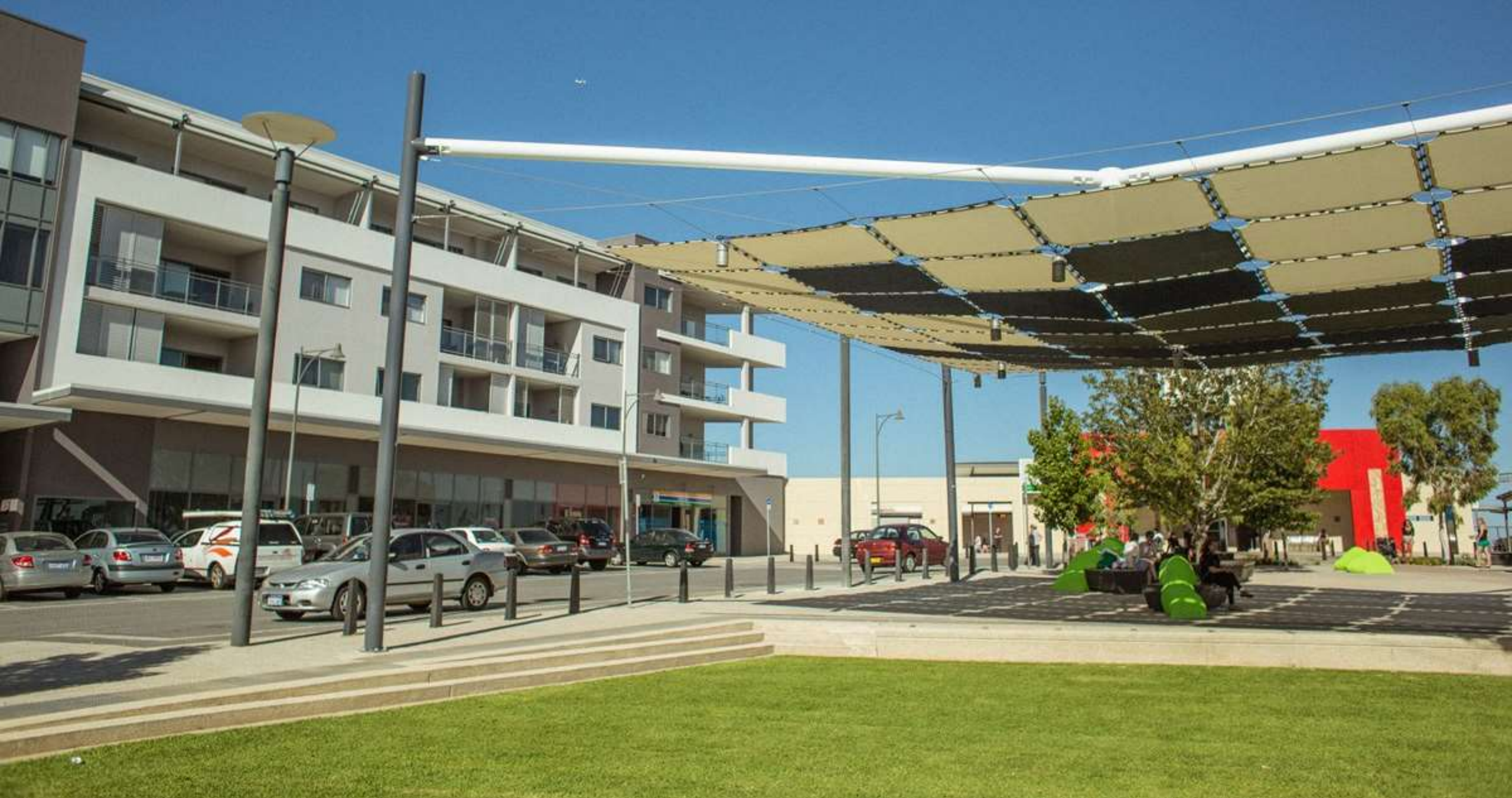
Cockburn Central Station, Perth
